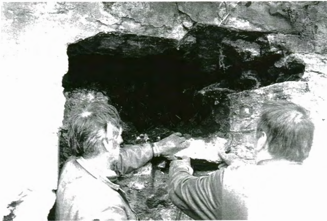
Fig. 7 Removal of inner blocking in progress.
