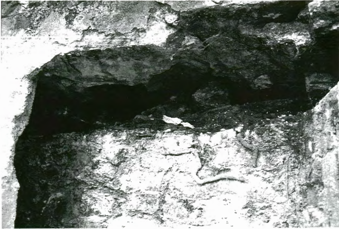
Fig. 6 Wooden lintel above inner blocking.
