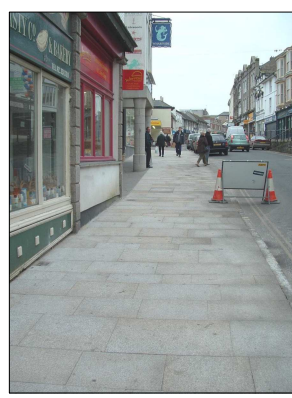
Example of recently paved granite footway in Penzance
